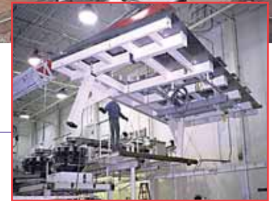
Modular panel being lifted into place; shortened installation to only 7 days.
