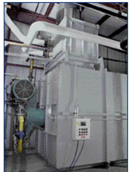
*The Booster Heater mounts over the exhaust stack of most any heat exchanger. It extracts heat from exhaust gases to preheat cooking oil before it enters the heat exchanger.*
